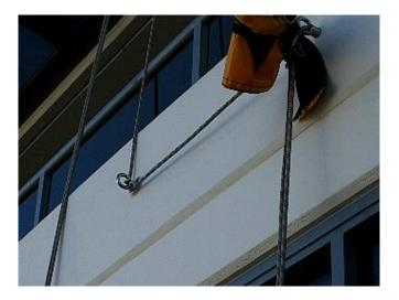
Close up clearly showing backup rope behind adjacent deviation anchor
