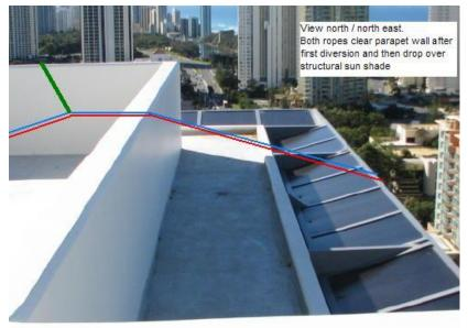
7. After Operator A had installed his diverted ropes (over the edge), Operator B (on the roof) then connected himself to both main and safety and negotiated the parapet wall and sunshade, installing edge protection and joined operator A to start cleaning.
